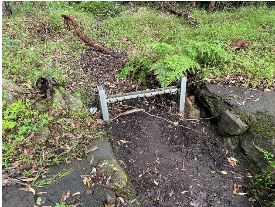
Figure 11: Full gross pollutant trap below Britannia Street
