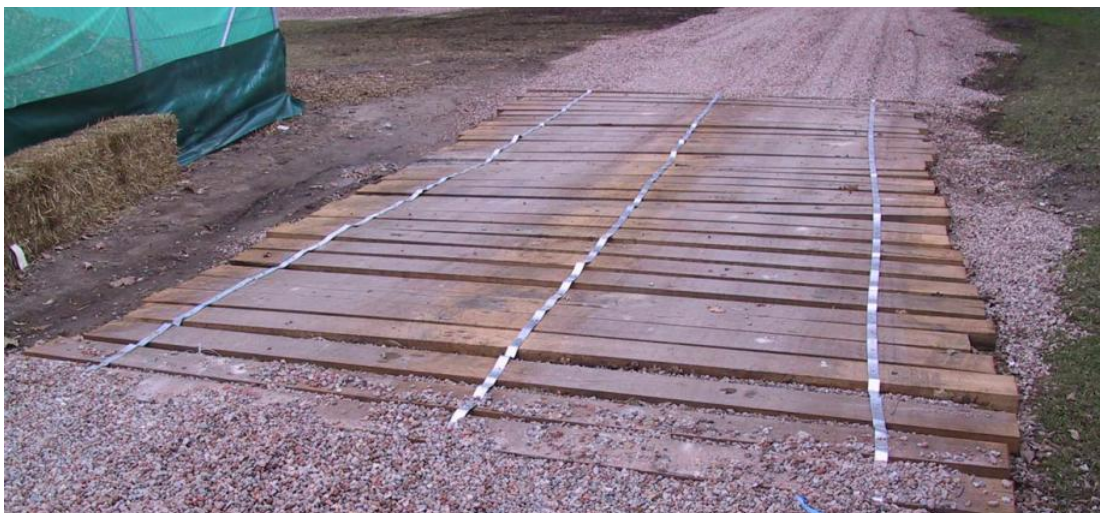
Figure 23 – Example of acceptable Tree Protection Area ground protection. (Image: Arterra)
